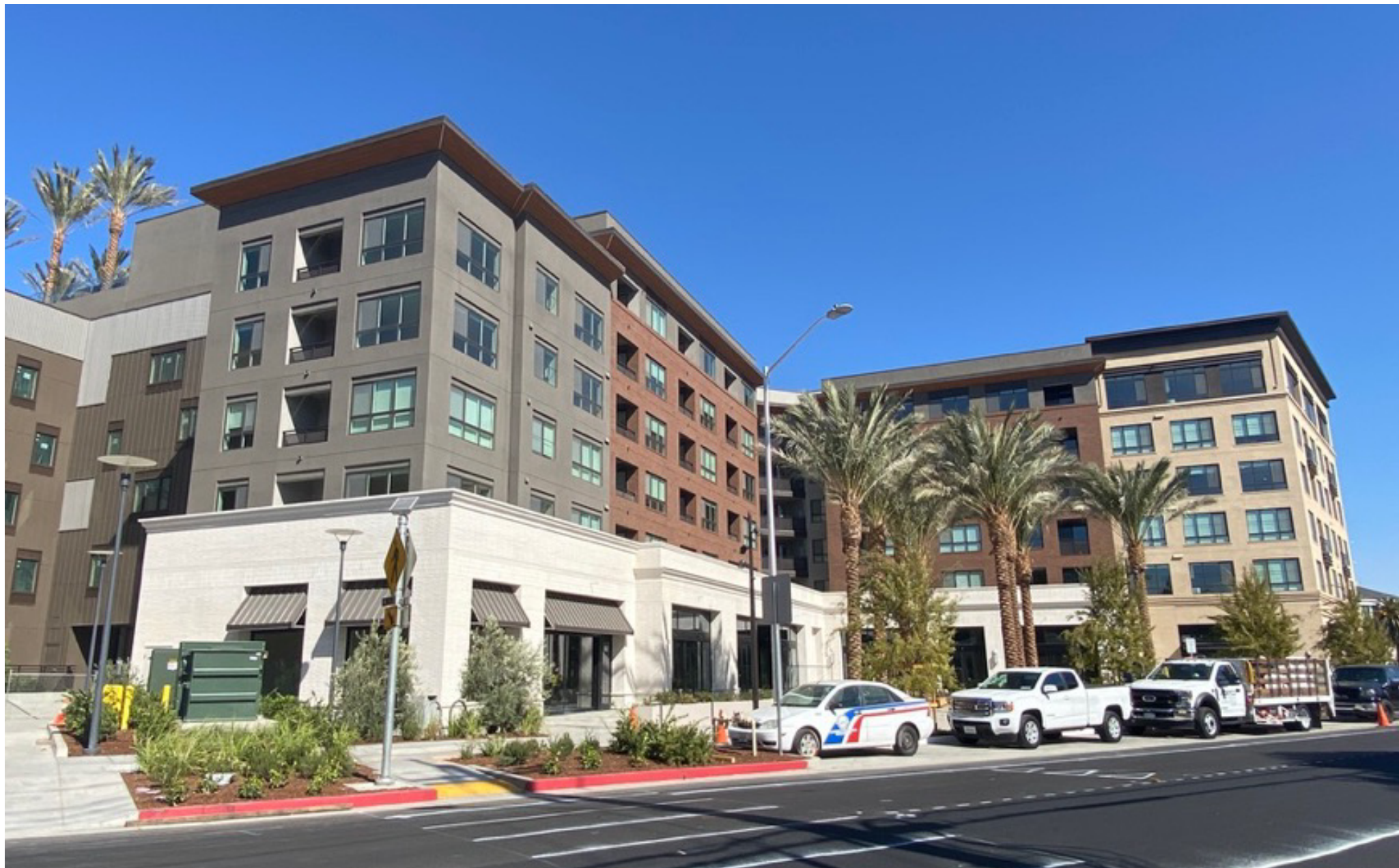
The Benton in Santa Clara along the ECR replaces a long-term storage facility
